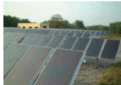
Figure 9: Thin-film PV arrays in New Delhi
