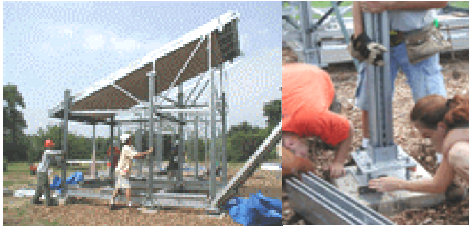
Figure 11: installation of ground-mounting structures at Austin (Texas)
