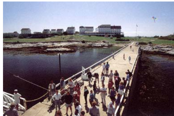
Figure 37: Star Island’s wharf
